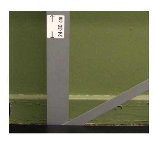
The bottom bracket must fall within the 24-30 cm range from the ground.
